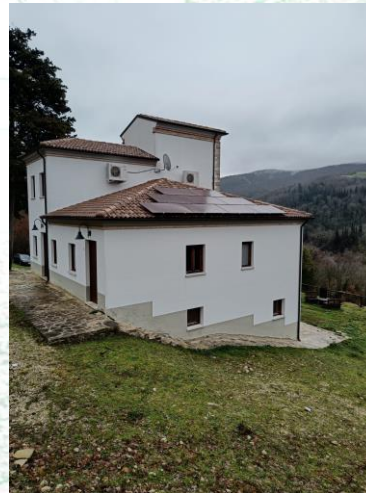
First solar plant: January 2023
